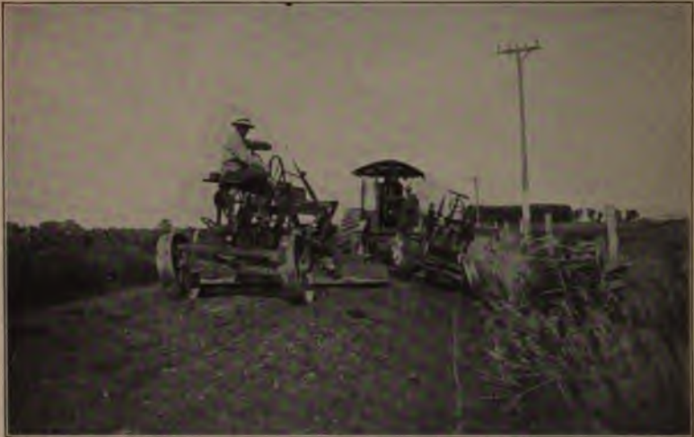
Two Reclamation Graders on Road Construction. Figure 15.
